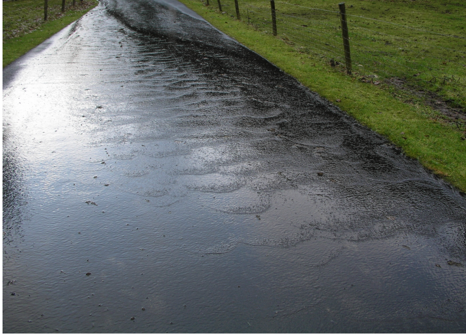
Figure 22: Roll waves on an asphalt road in the rain (Image copied from http://www.maths.ox.ac.uk/~fowler/pictures/gallery.html ).
